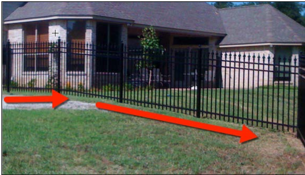
Figure 19 - Aluminum Fence Panels Racked to Follow Grade Down
