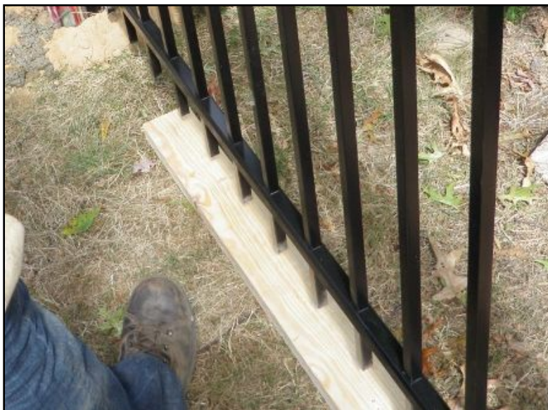
Figure 12 - Use a Piece of Wood Under Your Fence Panel to Preserve Your Desired Under Panel Gap
