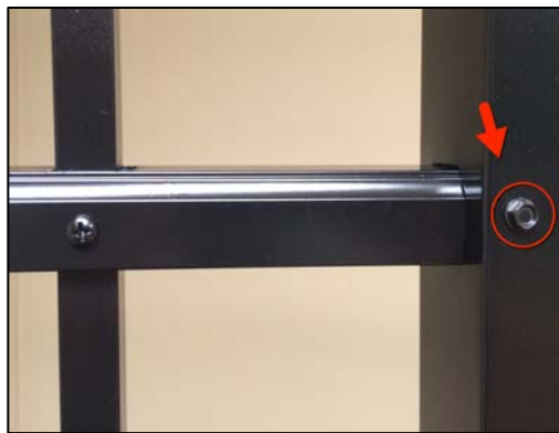
Figure 13 - Self-Tapping Screw Installed Into Post and Rail
