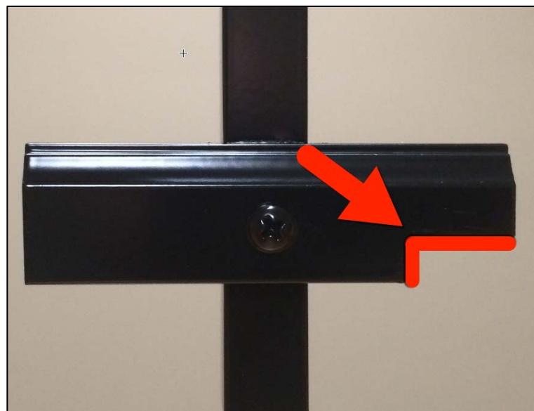
Figure 17 - Notch Lower Portion of the Cut Rail 3/4" x 1/4"
