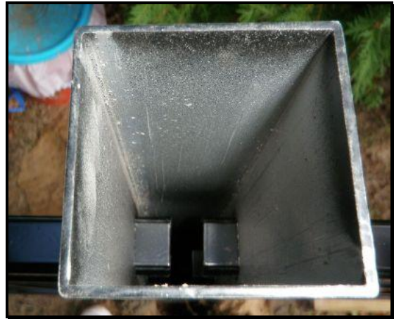
View from top of line post showing rail installed
