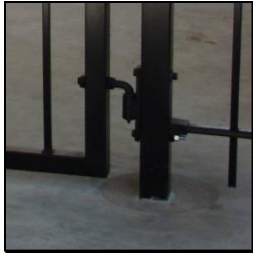
Core Drilled Post
