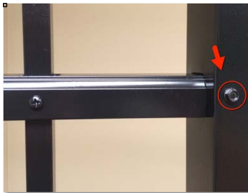
Figure 13 - Self-Tapping Screw Installed Into Post and Rail
