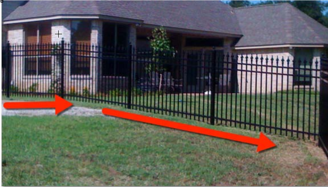
Figure 16 - Aluminum Fence Panels Racked to Follow Grade Down
