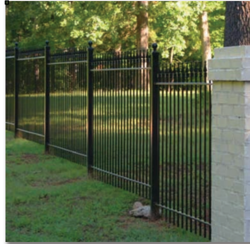
Figure 12 - Stair Stepped Fence Panels
