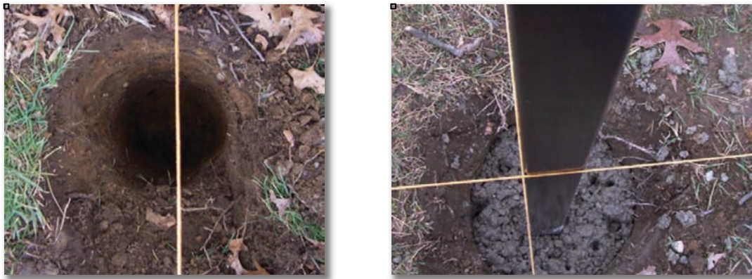
Figure 6 - Post Hole Should be Positioned so That The Centered Post Will Contact Your String Line
