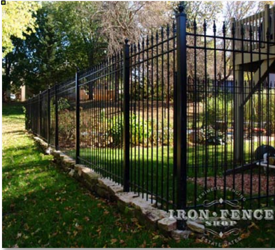
Figure 11 - Backfilled with Stones
