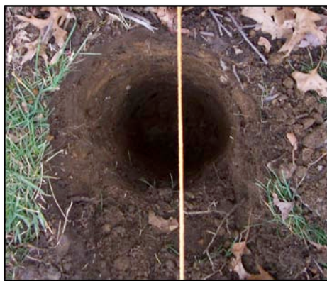
Figure 5 – Running a String Will Also Help Keep Your Post Hole Centered
