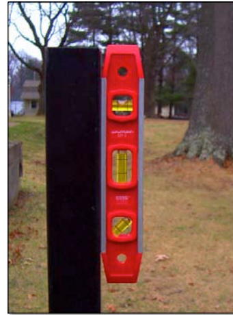
Figure 7 - Be Sure to Check Level as You Proceed
