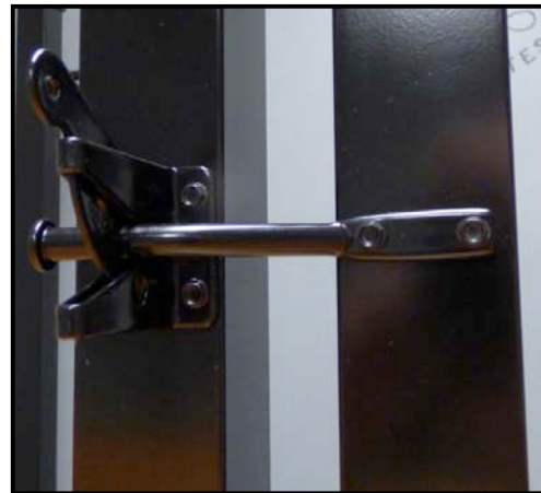
Figure 26 - Latch on Post (left) Arm on Gate (right)
