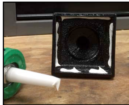
Figure. 21 - Apply Under the Cap
