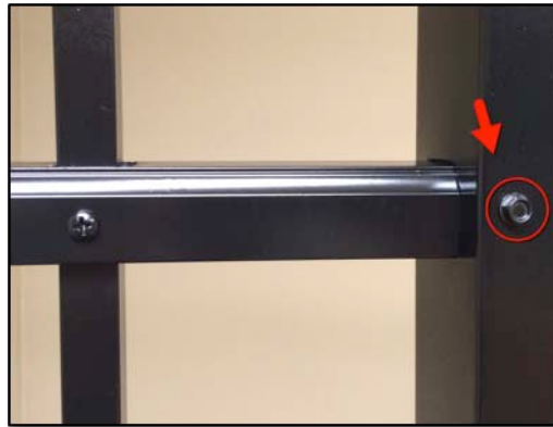
Figure 13 - Self-Tapping Screw Installed Into Post and Rail
