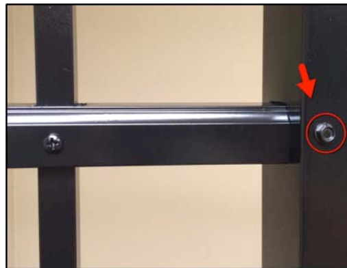
Figure 13 - Self-Tapping Screw Installed Into Post and Rail
