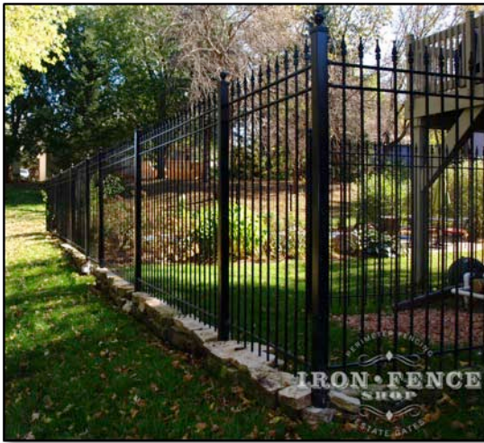
Figure 12 - Backfilled with Stones
