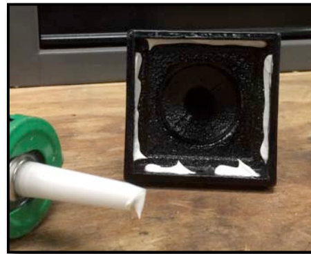
Figure. 15 - Apply Under the Cap
