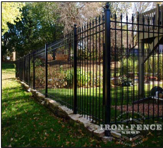
Figure 12 - Backfilled with Stones
