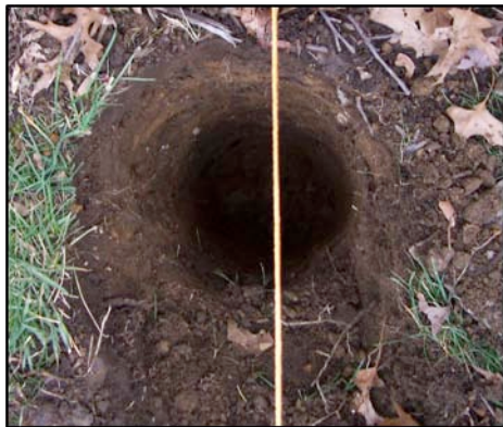
Figure 6 - Post Hole Should be Positioned so That The Centered Post Will Contact Your String Line
