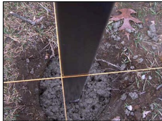
Figure 6 - Post Hole Should be Positioned so That The Centered Post Will Contact Your String Line
